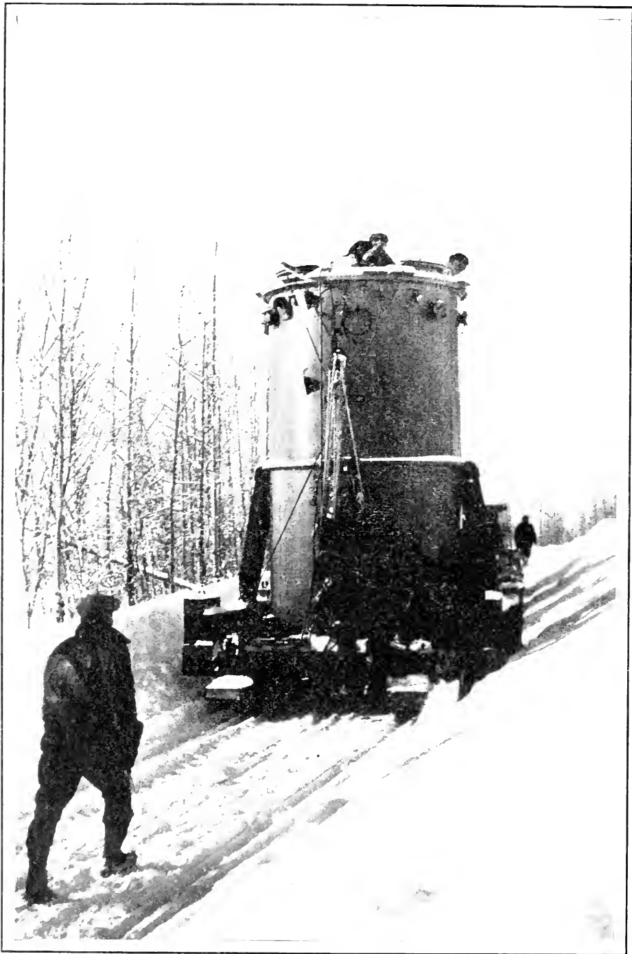
POWER FOR THE GOLD MINES OF NORTHERN ONTARIO Transportation Difficulties Overcome—Twenty-six Miles by Tractor Transformer of 1,500-kv-a. capacity en route to Matachewan
